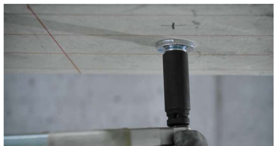
Step 14: Installation of the Hilti filling set manually or using the SI-AT-22 Adaptive Torque Module, ensuring all components are considered and the maximum torque is observed.
