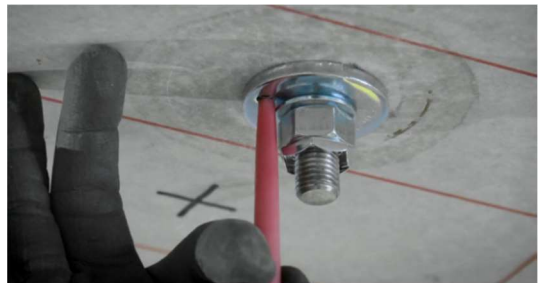
Step 16: Filling the Hilti sealing disc with suitable Hilti injection mortar using 1–3 strokes, as specified in the installation instructions.
