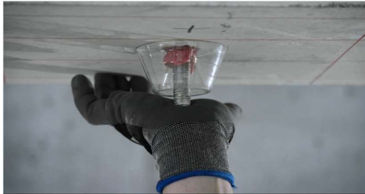
Step 11: Inserting the threaded rod to the bottom of the drill hole, followed by a visual inspection to confirm that a sufficient amount of mortar is visible at the drill hole opening.
