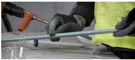
Step 7: Preparation of the threaded rod with Hilti drip plate HIT-OHC2.
