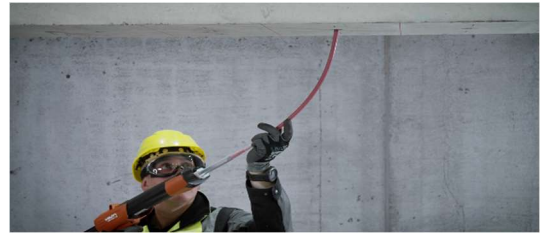
Step 10: Injection of the drill hole from the bottom up within the working time using appropriate accessories to ensure bubble-free filling and sufficient mortar quantity.
