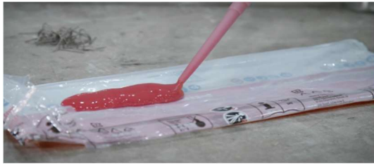
Step 9: Discarding the first strokes as specified in the installation instructions to ensure proper mixing of resin and hardener.
