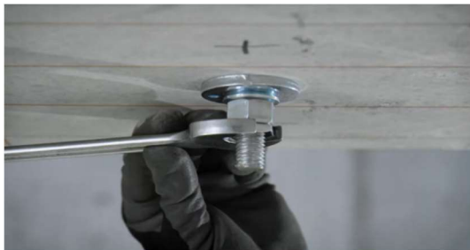
Step 15: Tighten the lock nut hand-tight.
