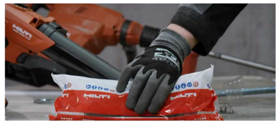
Step 8: Preparation of the specified injection system, including all required accessories.
